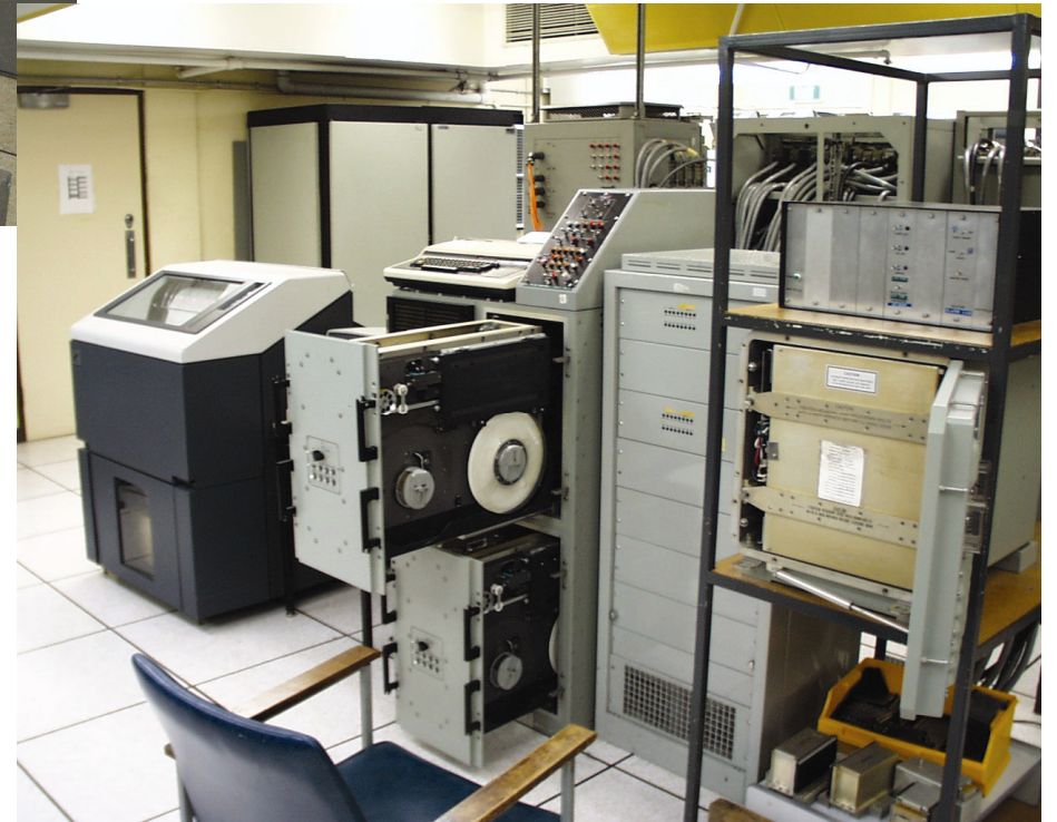
An OJ-172 DEAC in the DDG equipment room
