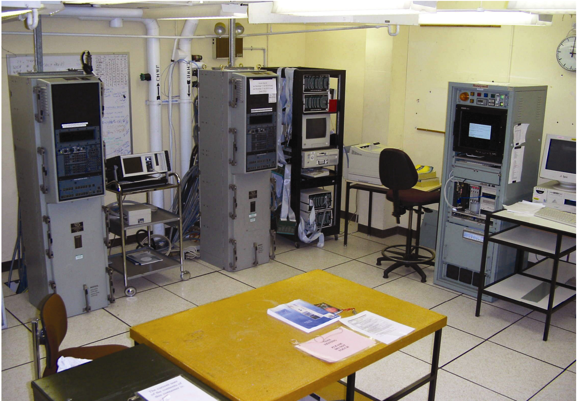
FFG equipment room, 2004
