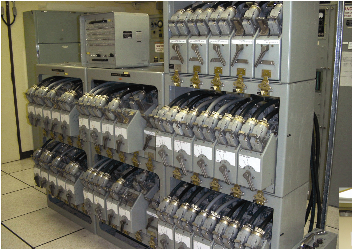
Banks of 1299 switches for FFG suite and MTS – everything could be connected
