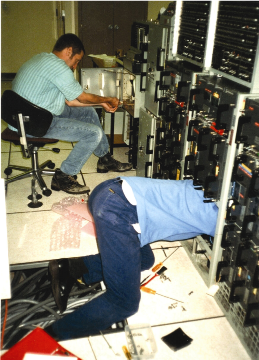
AN/UYK-7 in DDG equipment room
