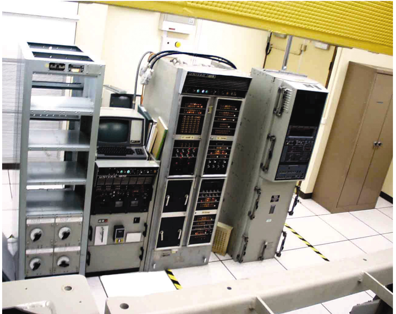
The new and the old – AN/UYK-43 (right), next to DDG Mk152 fire control computer
