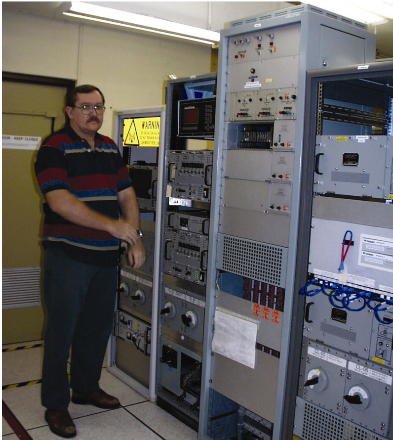
Graeme Ward at Link-11 Data Terminal sets
