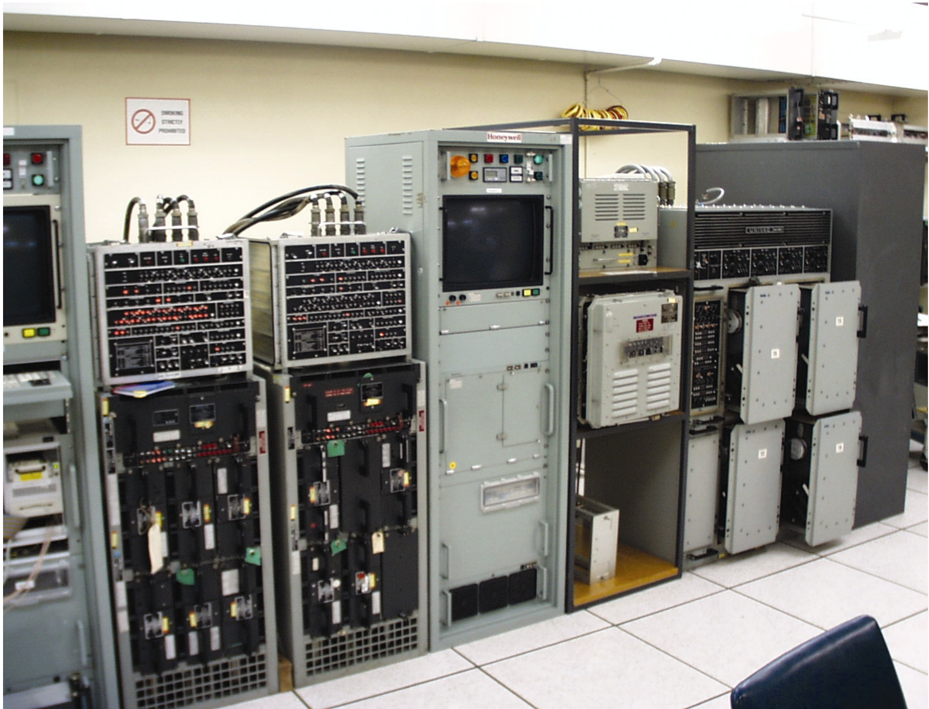
Rear wall of DDG equipment room, 2004
