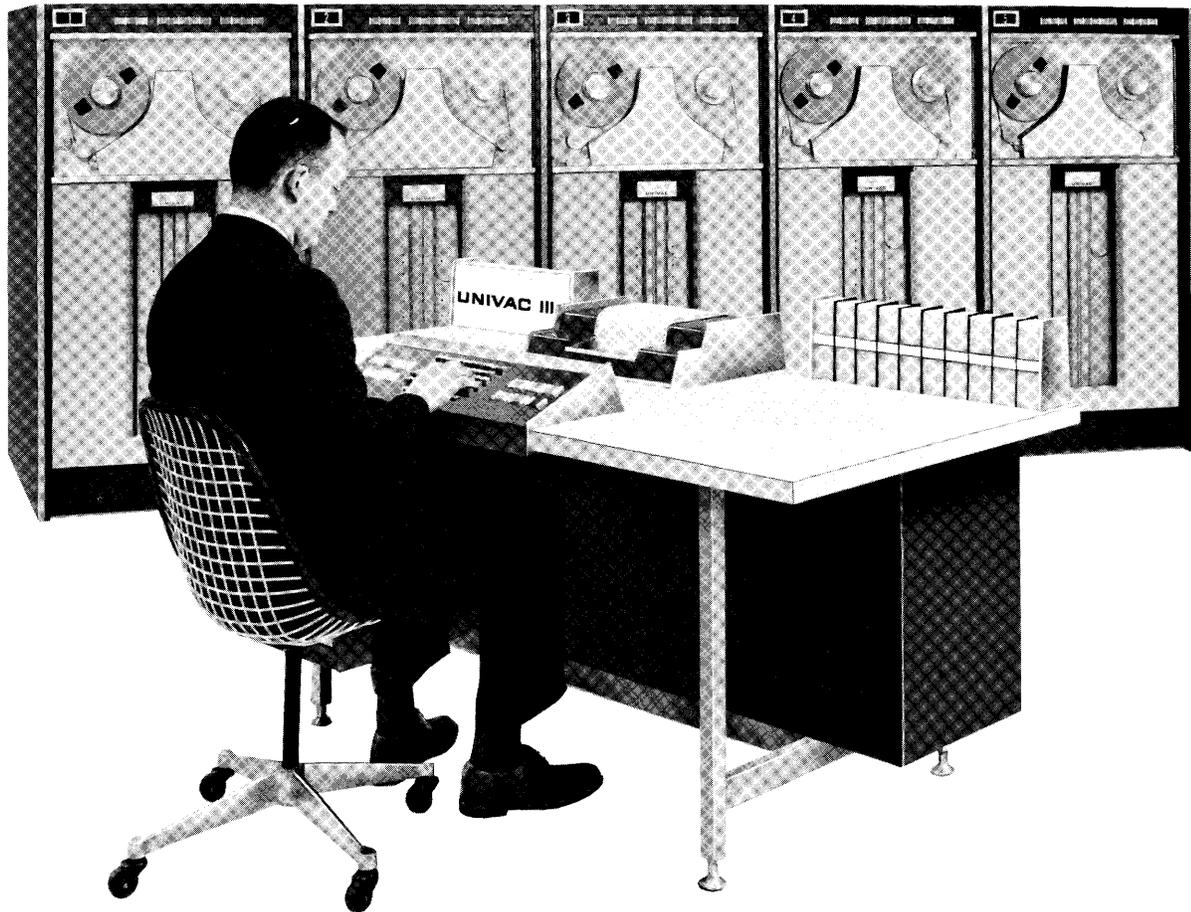
A typical basic UNIVAC III System comprises a Central Processor with magnetic-core storage, a UNISERVO IIIA tape system, a High-Speed Reader, a Card-Punch Unit, and a High-Speed Printer. The basic system may be expanded to include up to 32 UNISERVO IIIA tape units, a UNISERVO IIA tape system, and a variety of peripheral units, as shown in figure 1-1.
