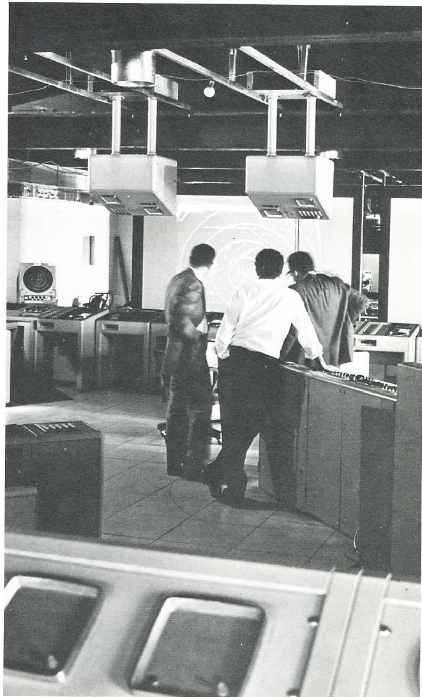
High-speed digital data processing equipment will play an important role in the New York Common IFR Room which is shown in the photo while equipment was being installed and tested during October. The two large-screen displays (one shown illuminated in the photograph) and eight display consoles provide a composite picture of sensor video and the computer-processed alphanumeric information.
