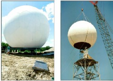
Above: Two pictures of the WSR-88D NEXRAD system being installed in Chanhausen, MN, in 1994. The project was headed up by the Great Neck, NY, division of the company with several key portions of the system (including the digital signal processor) were designed in Fagan, MN.
