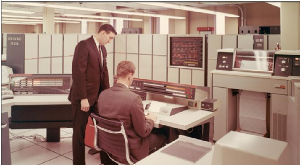
Below: The UNIVAC 1108 computer which was first delivered in late 1965. MAPPER software became a standard in later computers in the 1100 series and is still in use today by Unisys.
