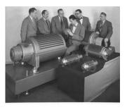
in the Washington DC CIA predecessor's facility in December 1950 – the world's first stored program computer installed into a customer's facility. The drums shown were the world's first production 'hard-drives.'
